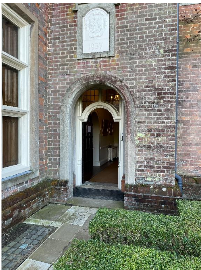
The accessible entrance to the property located on the North Front
